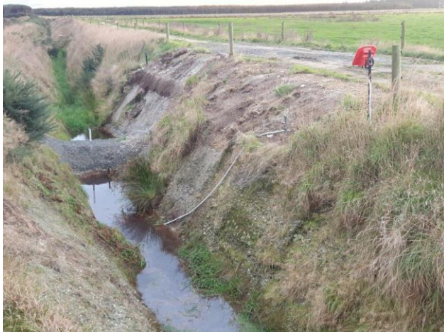
Figure 11: Site 1 Gravel weir initial installation looking upstream, May 2021.
