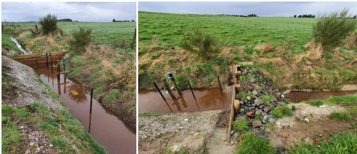
Figure 9: Site 4 Wooden weir looking downstream (left) and showing rock backfill downstream (right).
