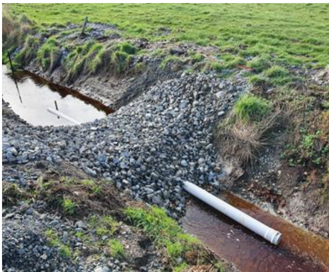
Figure 15: Site 3 after instatement utilising rock ballast (22 July 2021).
