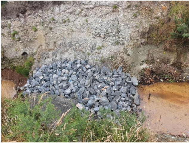
Figure 13: Reinstatement of Site 1 utilising rock ballast.
