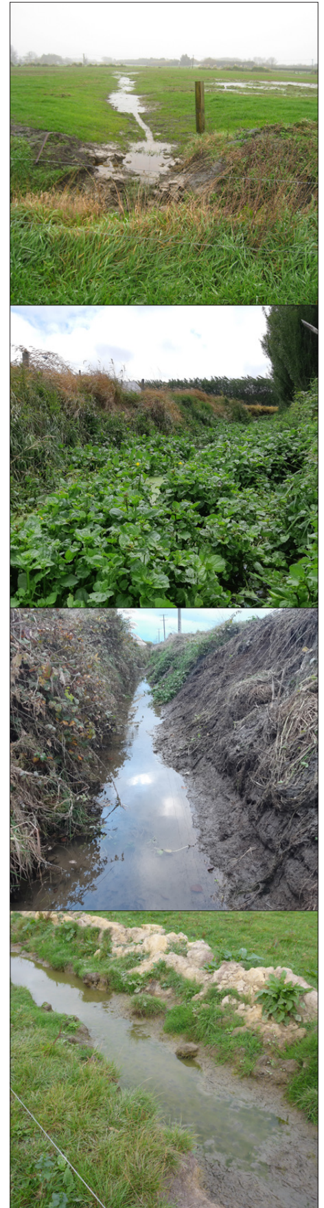
Figure 2. The issues raised in preliminary discussions were (A) flooding, (B) macrophytes, (C) drain cleaning, and (D) excessive fine sediment.
