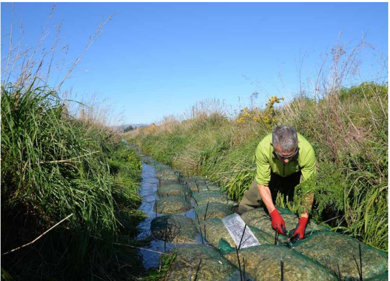
Installing a woodchip bioreactor on-farm.
