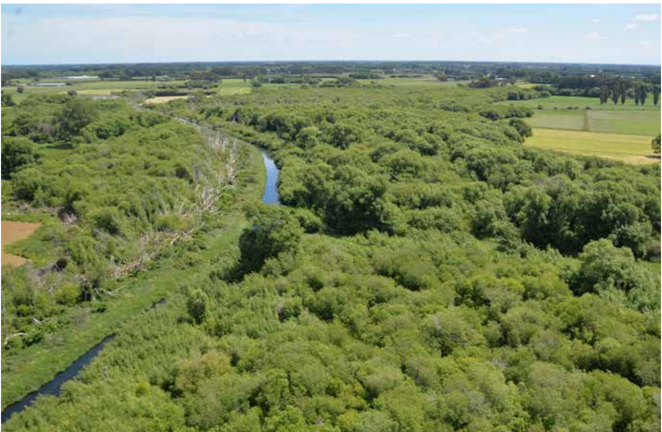
Tārerekautuku/Yarrs Lagoon, with willow control underway.
